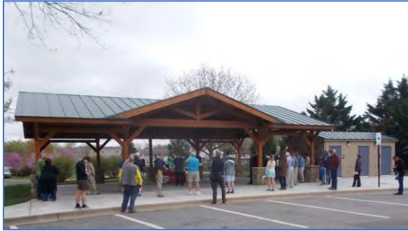
Front Royal's New Downtown Pavilion & Restroom Constructed with Local and Grant Funding
